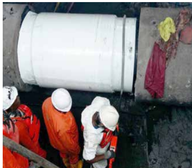
•Holiday detection of repaired joint
