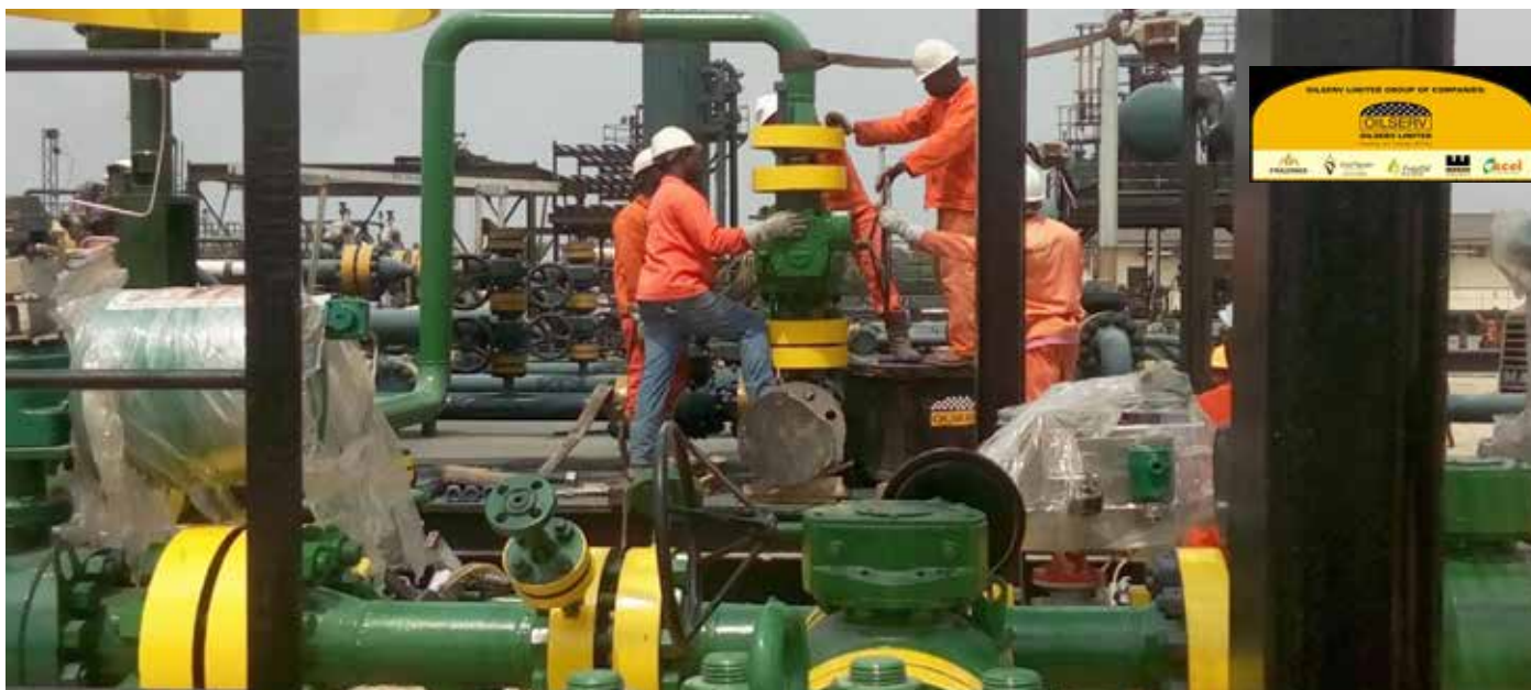
•Hook-up to existing 6" inlet line
