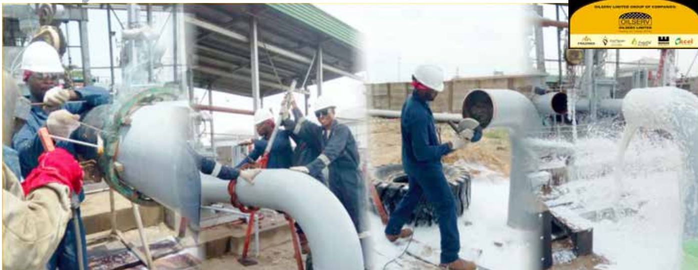
•Pipe tie-in, cold-cutting, pipe smoothening using grinding machine, and neutralizing PMS environment using form compound
