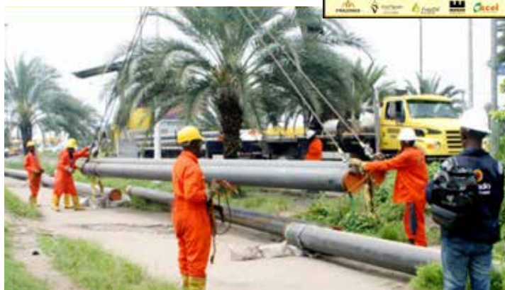
• Offloading and stringing of 3LPE coated linepipes along the right of way
