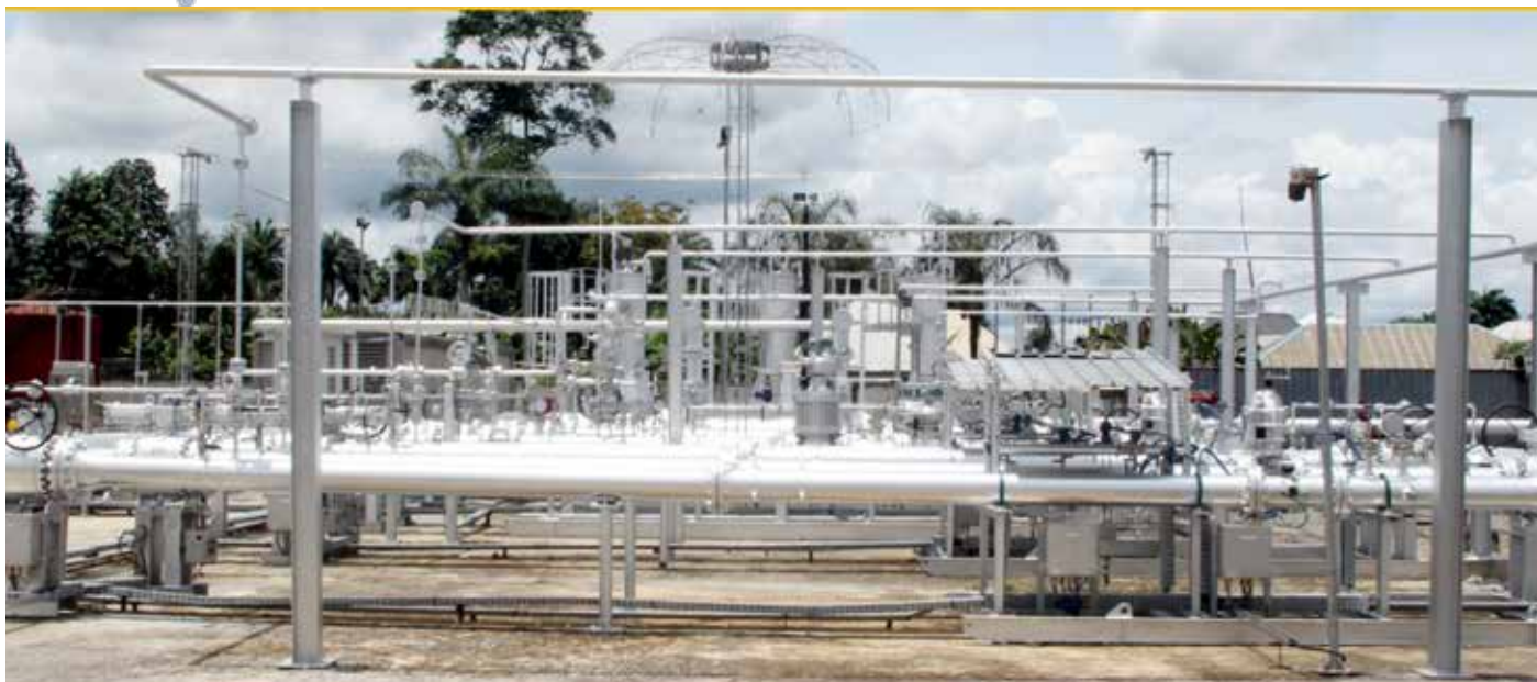
•Pressure reduction metering system facility
