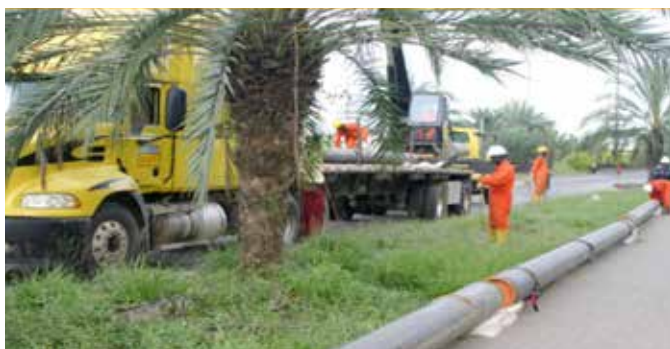
• Offloading and stringing of 3LPE coated linepipes along the right of way
