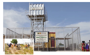
Completed 5000 gallons Solar Hybrid System Powered Water, Sanitation and Hygiene facility provided by NNPC/SNEPCo as part of its humanitarian intervention in Kwana Local Government Area of Borno State. Project was completed in 2020 serves over 11,450 people resident in Kwaykassar community.
